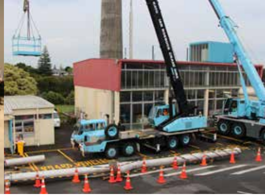
New chimneys going up
